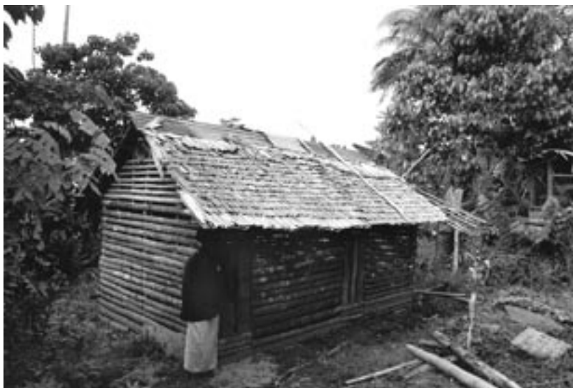
A kokorako house at Sasamuqa village, Choiseul Province, Solomon Islands. The house is made of timber slats that make it strong enough to protect the kokorako against dogs. The roof is palm leaf.
