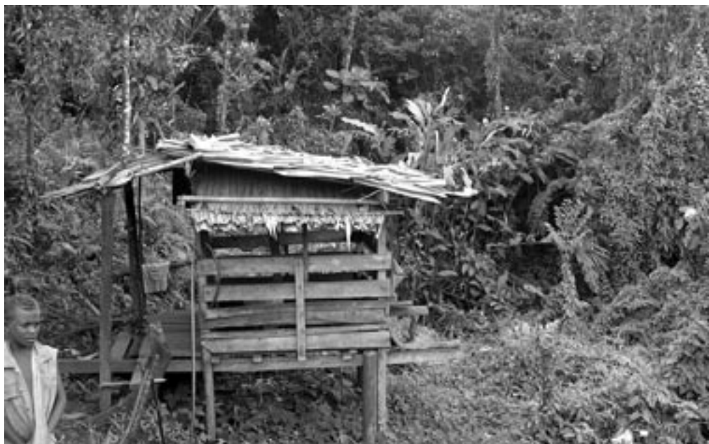
A pig house with a leaf roof and strong walls made of wooden planks. Photo: T. Jansen
