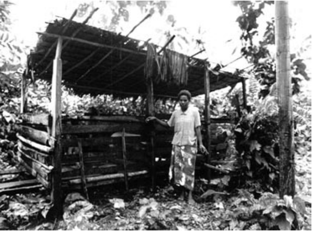
Rose Adewane with one of her pig houses. The houses have slatted floors, the frame and sides are made of cut timber and a leaf roof shelters the pigs from sun and rain.
